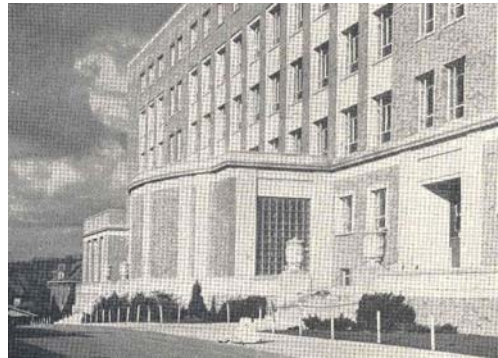
Mineral Industries Building, also known as White Hall, was dedicated in 1942 and housed the School of Mines and College of Mineral and Energy Resources until 1990.
