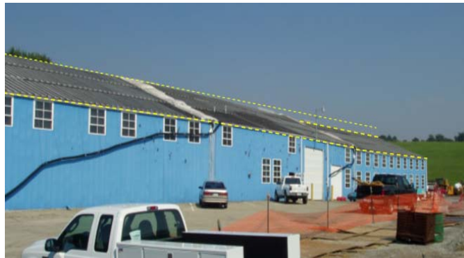
The longwall subsidence influences on this 250-ft long, 60-ft wide and 30-ft tall industrial building were successfully mitigated with a number of innovative methods. The longwall mining operation was conducted about 300 ft below this building. The business inside the building was not interrupted by the subsidence event.
